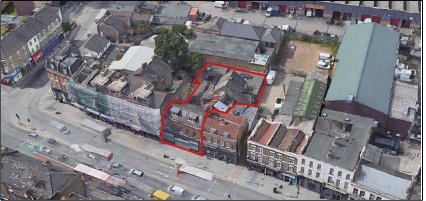
The site – frontages on to High Road and Percival Court
